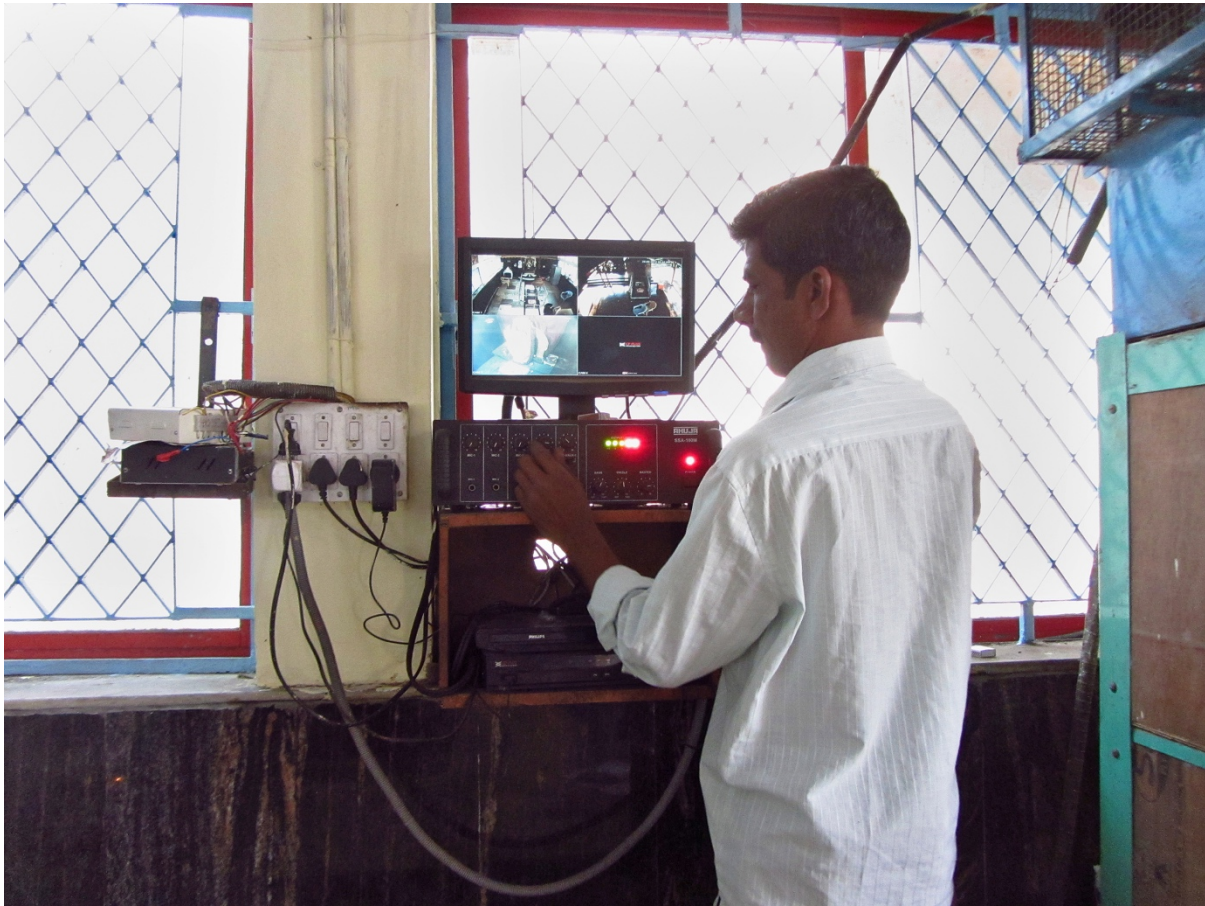
Figure 3 Documentation still from the 2014 performance of CFTS. Photo: Ishan Gupta
